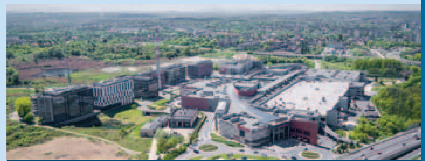
Bonarka City Center and Bonarka for Business office complex, Krakow
