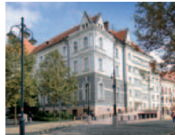
Functional Extension Town Rehabilitation, Kaposvár
